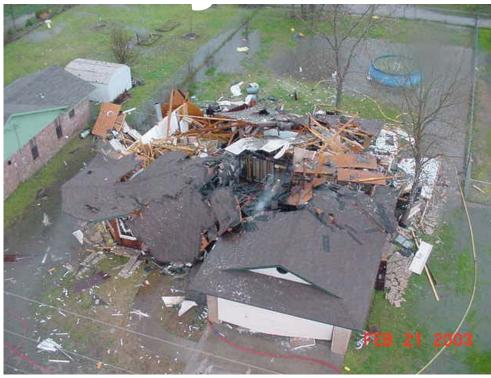
Gas related damage to a home in Texas. This is the type of damage that can result when lightning arcs and travels on CSST
